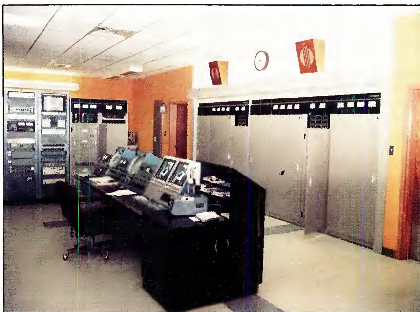
A 120kW Klystrone transmitter installed at WCLP-TV Channel 18 in Chatsworth, GA. (Courtesy of Comark.)
